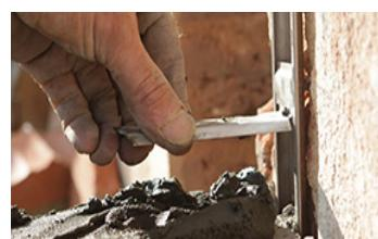
A stainless steel system, designed to join new walls to existing masonry, suitable for both internal and external brick or block walls.
